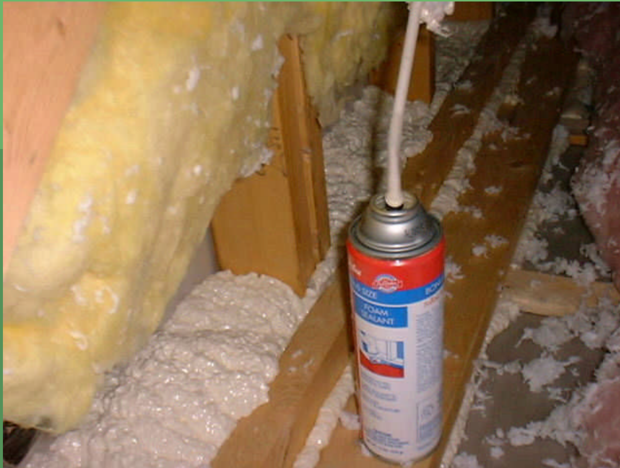
Foam airsealing installed at top of typical step-down wall in attic.
