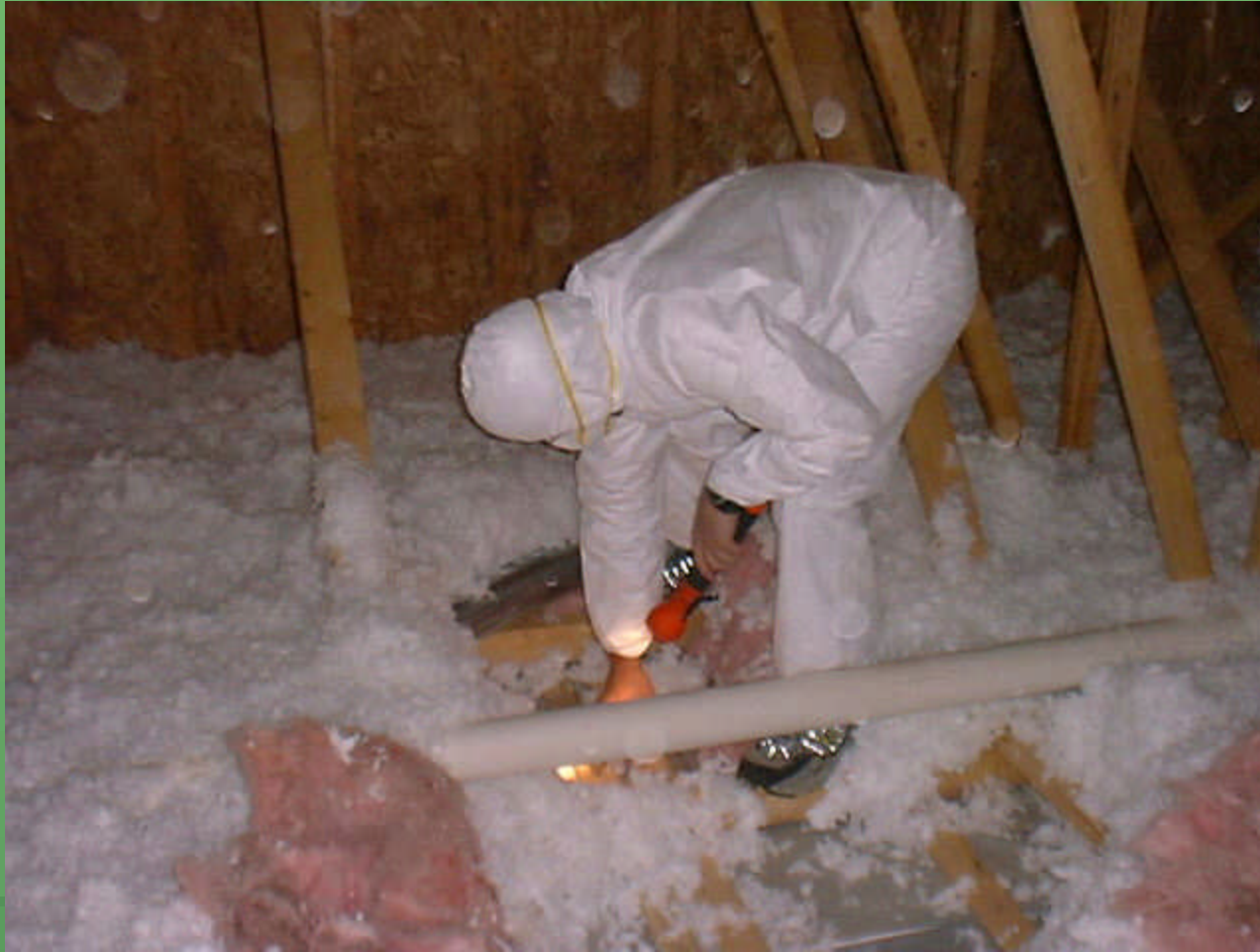
Using foam to air seal typical partition top in attic
