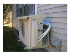
Outdoor component must be protected by a rain cap if located under a drip edge.
