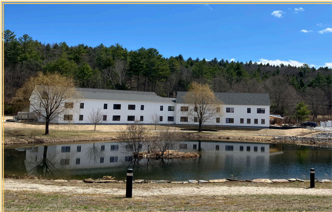
Edgewater Village, Farmington, Maine, a 25-unit affordable apartment project for older adults. MaineHousing contributed 4% LIHTC funding.
