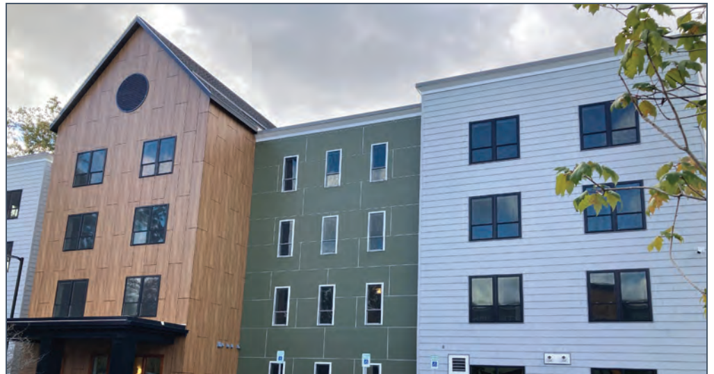
Lewis H. Emery Apartments in Westbrook, 30 new construction units for older adults, funded in part by the State HOME Fund.
