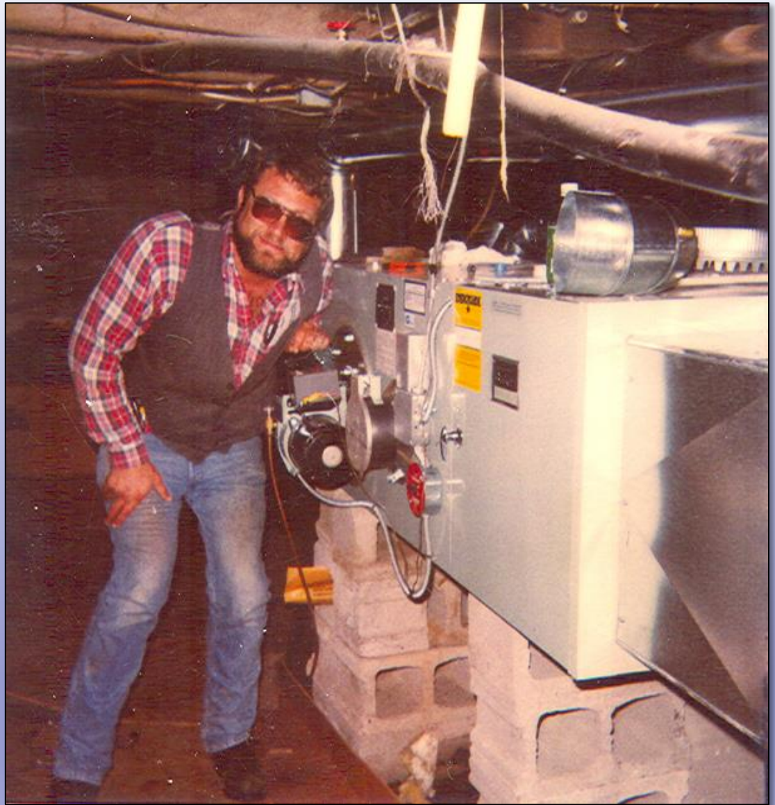
Mike Baran and a heating system.
