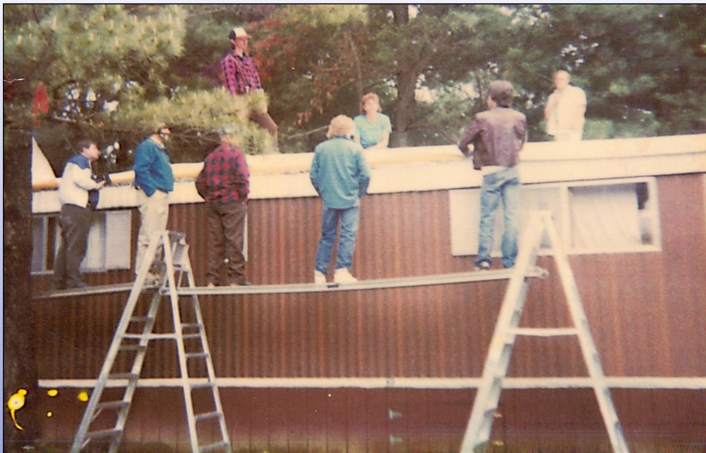
The 1988 New England Mobile Home Retrofit Conference in Lisbon, Maine, the Community Concepts crew demonstrates the installation of membrane roof.
